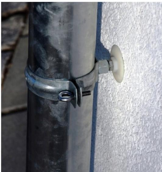
The patented IPL 95DS is delivered completely assembled; it consists of a one-piece plug including a sealing washer and a special threaded stud.
